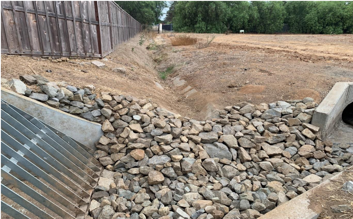
Photograph 14. Updated view of isolated disturbed wetland feature where rip-rap replaced southern cattail, facing west.
