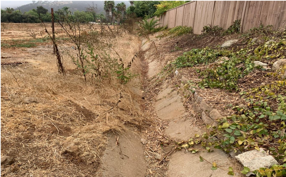
Photograph 15. Updated southeast view of project site and concrete v-ditch.
