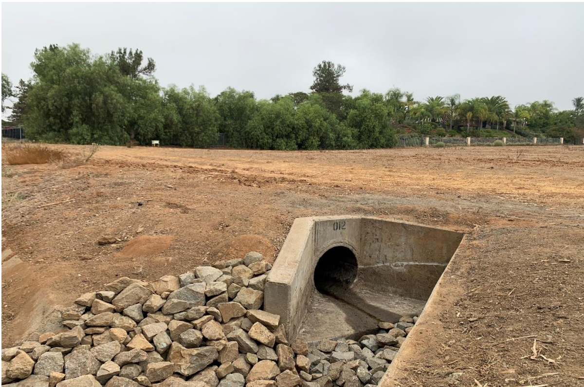
Photograph 16. Updated northeast view of project site, and underground culvert outlet.
