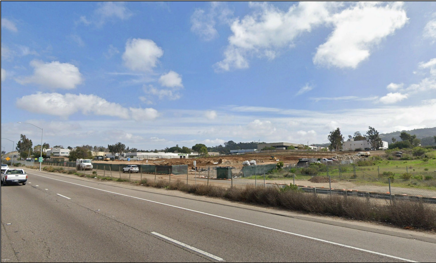
Figure 5a. Eastbound SR-78 (Existing View)
