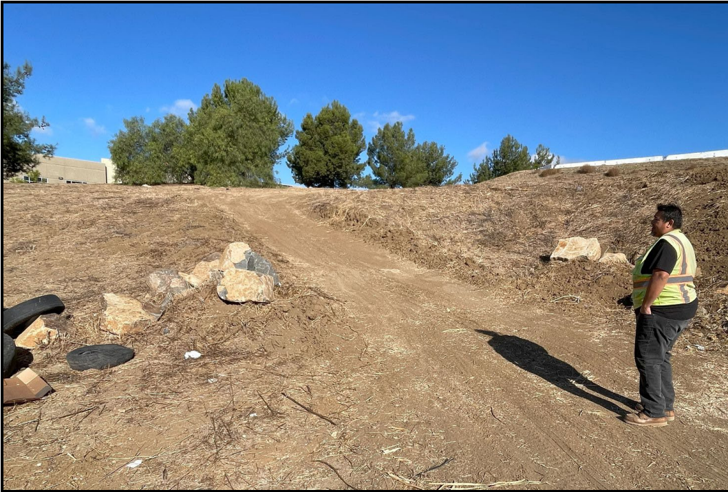
PHOTOGRAPH 8 Overview of Recent Cut-Graded Road, Looking Northwest
