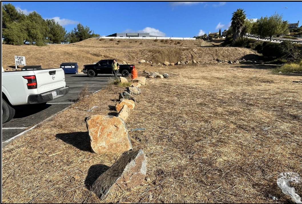
PHOTOGRAPH 7 Boulder Barrier East of Commercial Development, Looking North-Northeast
