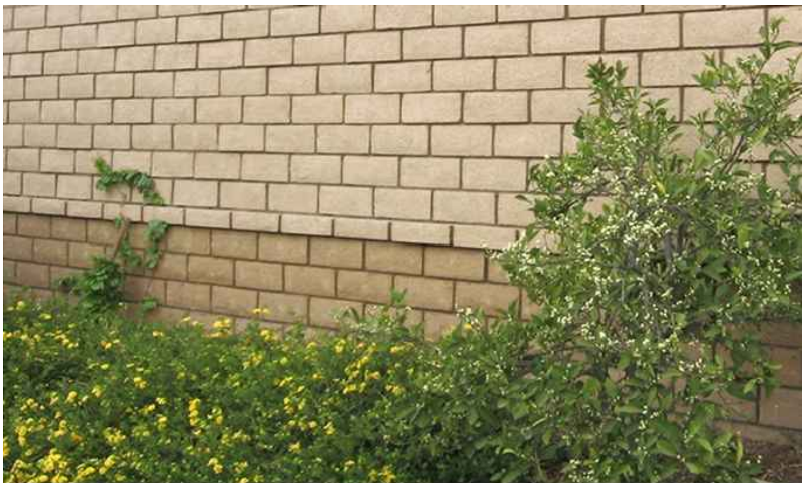
— Tan Slump Block Retaining Wall
