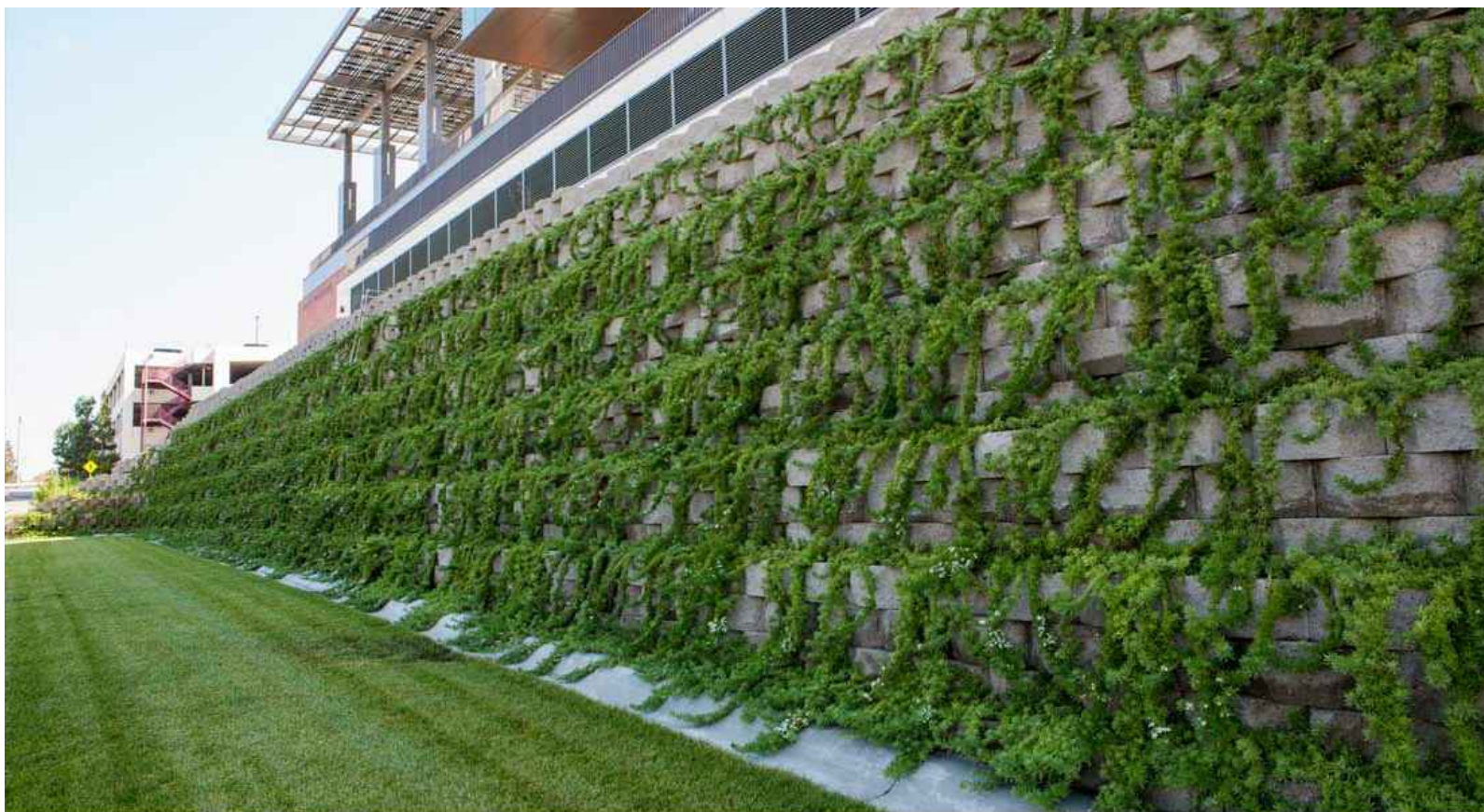
— Tan Geogrid Retaining Wall
