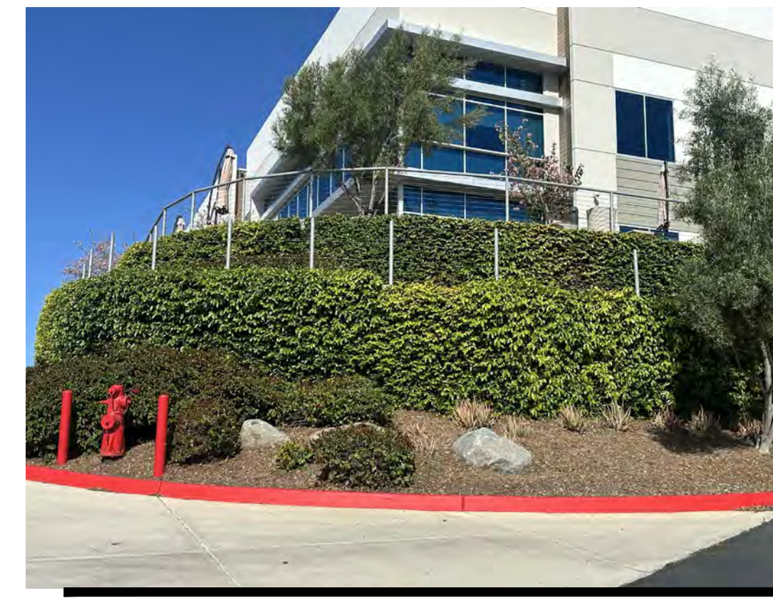
GEORGRID WALL PLANTED WITH VINES TYPICAL ILLUSTRATION
