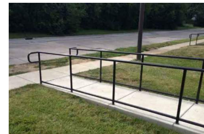
Ⓖ Ramp/ Stair Handrail
