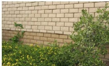
— Tan Slump Block Retaining Wall
