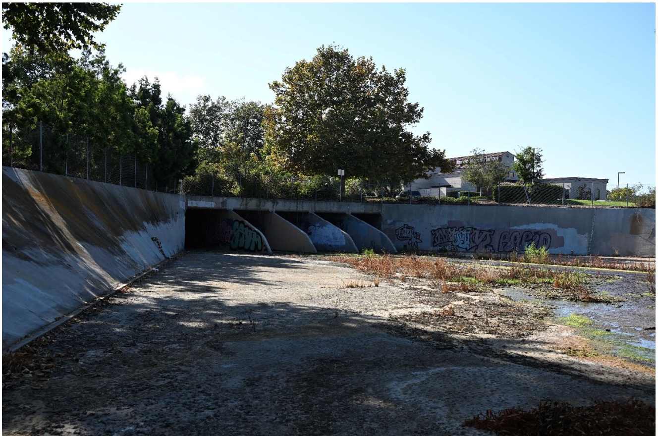
Figure 12. Concrete Transition Structure and Box Culverts below Reach 2
