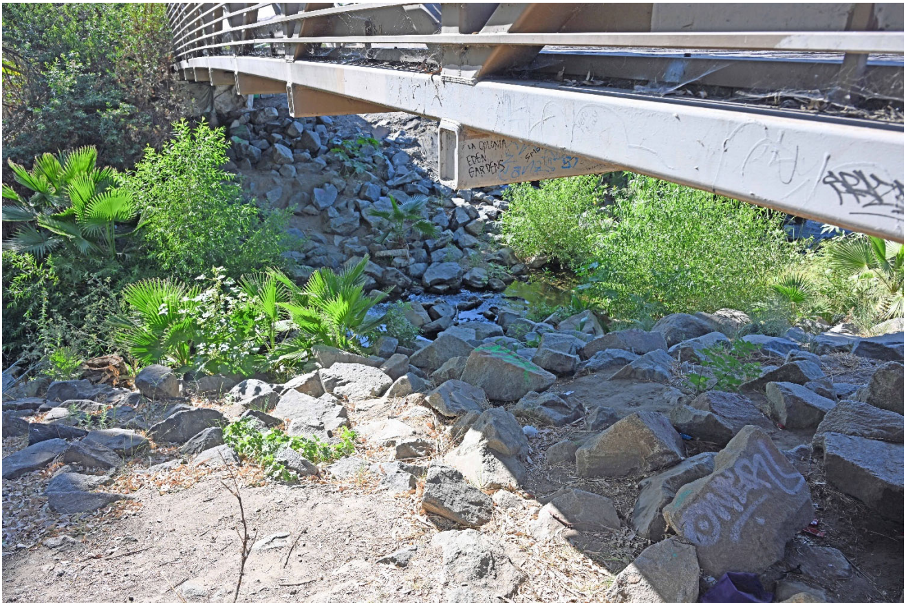
Figure 1. Riprap under Inland Rail Trail – Upstream End of Reach 1
