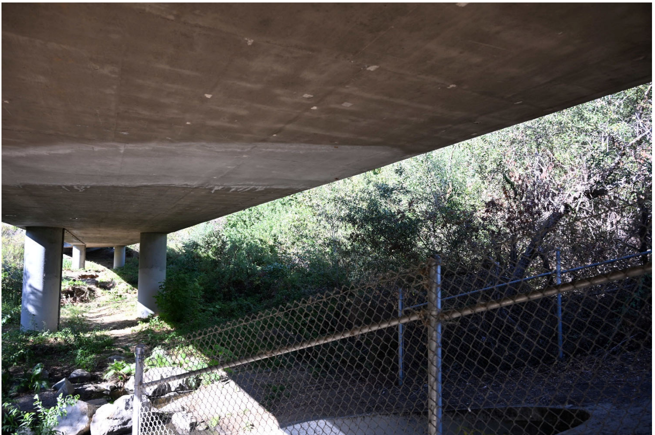
Figure 6. Reach 2 at Sprinter Rail Crossing - 84" RCP Outlet (POC) at Bottom of Figure
