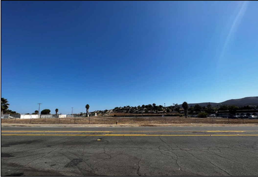
Figure 3.1-2. View 1 – From the South
