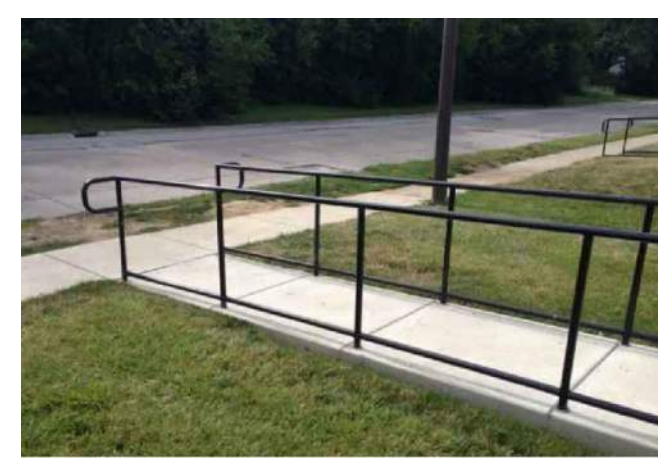
(G) Ramp/ Stair Handrail
