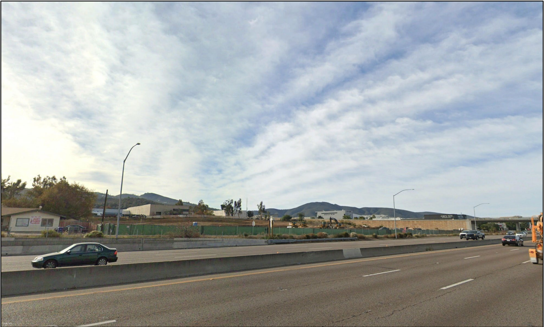
Figure 6a. Westbound SR-78 (Existing View)
