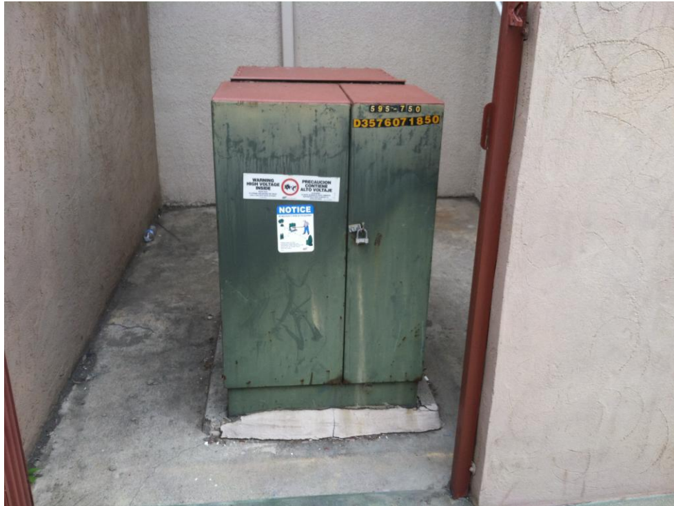
Photograph 15 – View of a pad mounted transformer, located adjacent to the swimming pool and associated storage shed.
