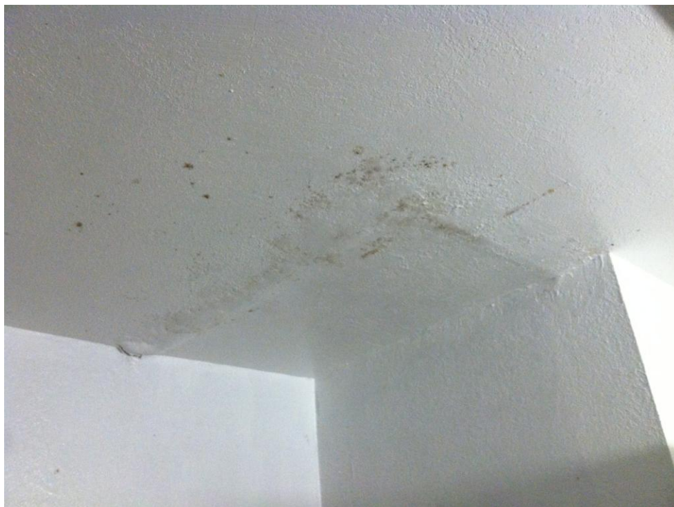
Photograph 22 – View of potential mildew residue found on the bathroom ceiling of Unit 111, located at 340 Marcos Street.
