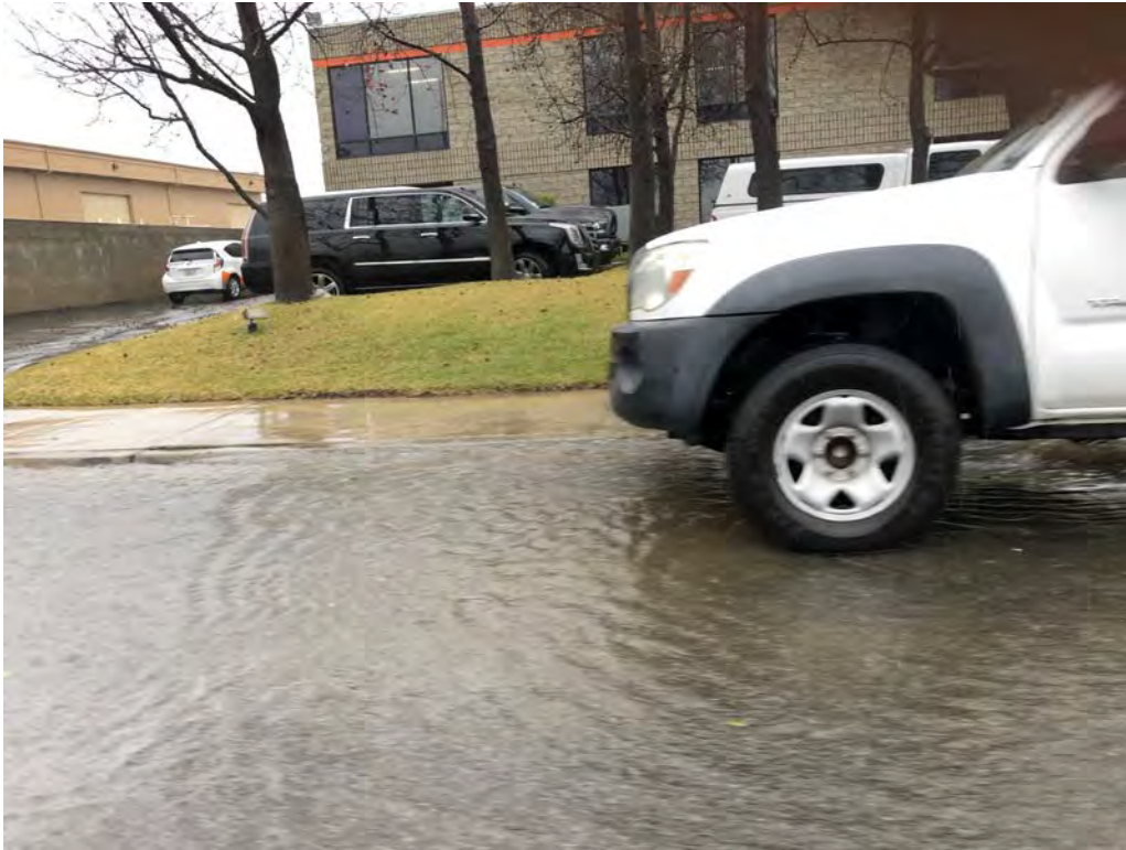
Figure 6-6: Runoff overtopping the curb along La Mirada Drive
