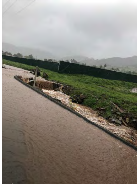
Figure 6-16: Surface conveyance via ditches along Mulberry Drive
