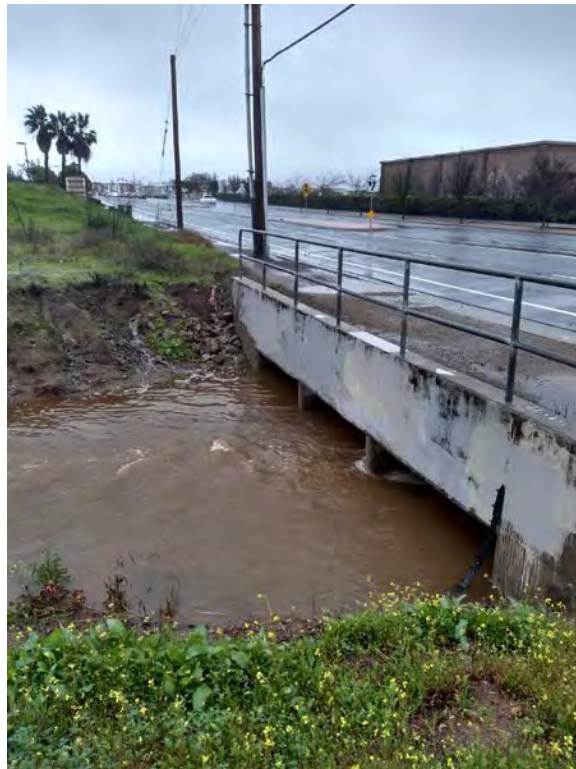
Figure 6-2 : Culvert across West Mission Road acting as a constraint
