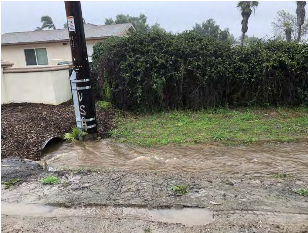
Figure 6-7: Surface flow via driveway culverts along Las Flores Drive
