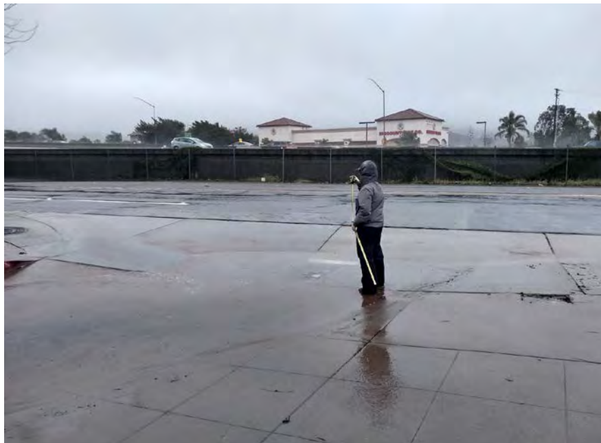
Figure 6-12: Flooding at the driveway crossing across Jerome's Furniture complex along Los Vallecitos Boulevard.
