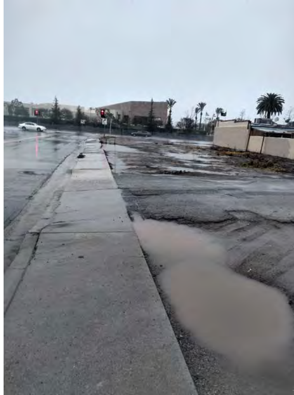
Figure 6-15: South of Firebird Lane at West Mission Road
