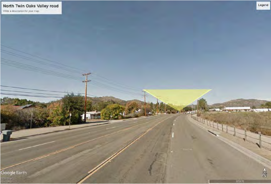
Figure 6-17: Google street view of North Twin Oaks Valley Road
