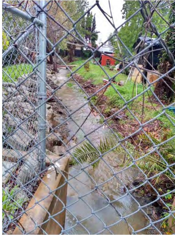
Figure 6-9: Existing Channel at South Santa Fe Avenue
