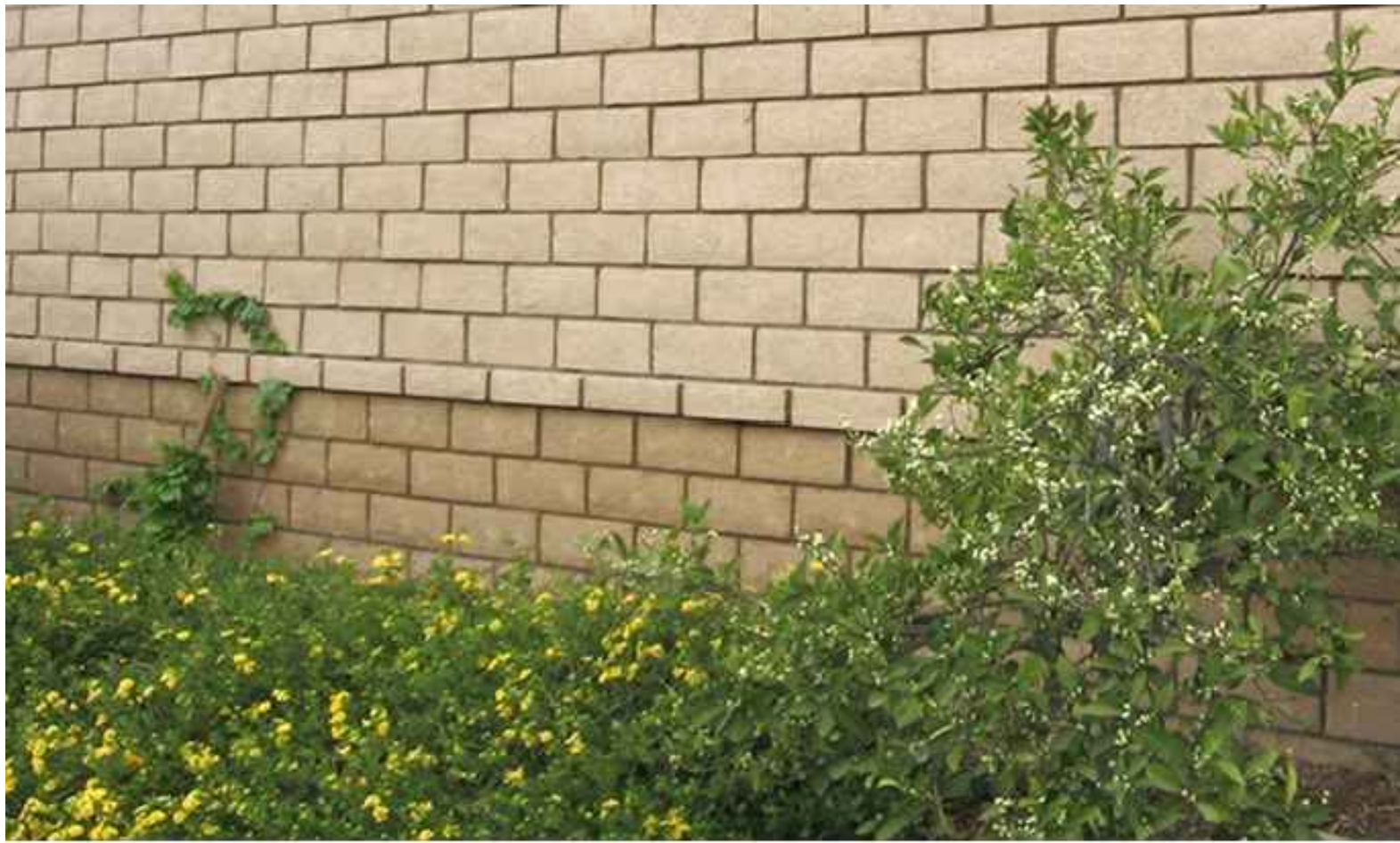
— Tan Slump Block Retaining Wall
