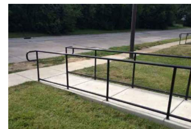
(G) Ramp/ Stair Handrail
