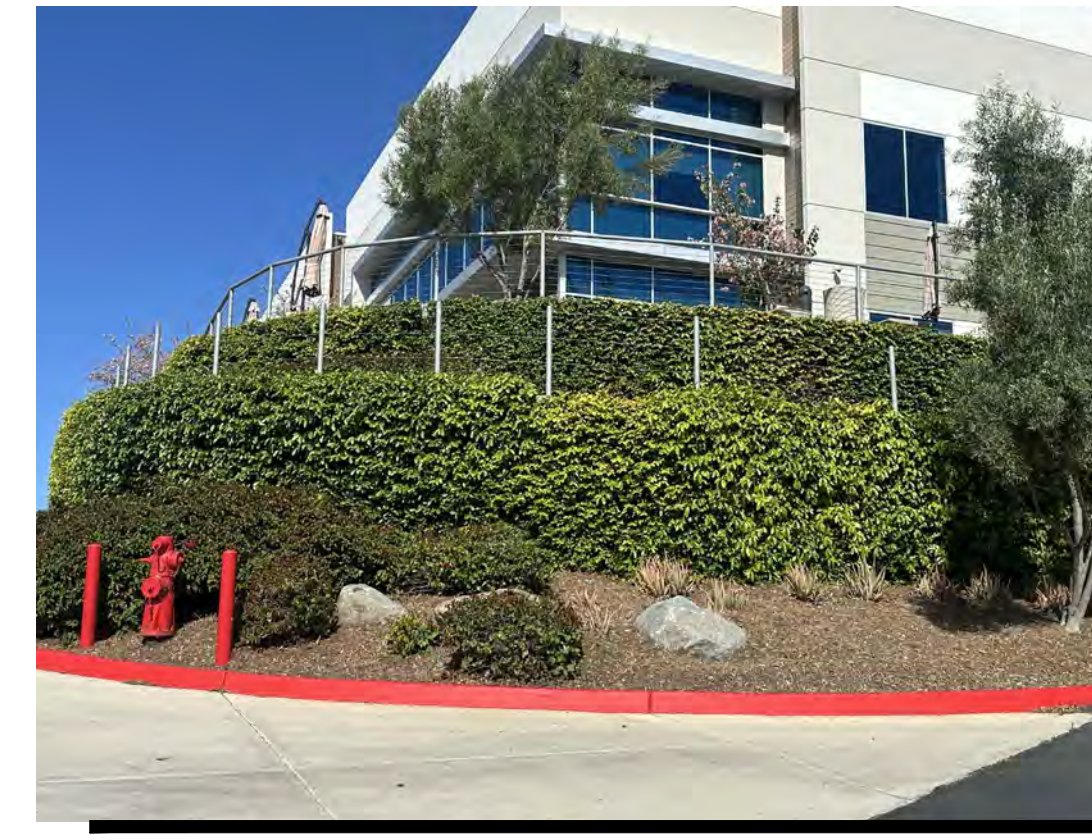
GEORGRID WALL PLANTED WITH VINES TYPICAL ILLUSTRATION
